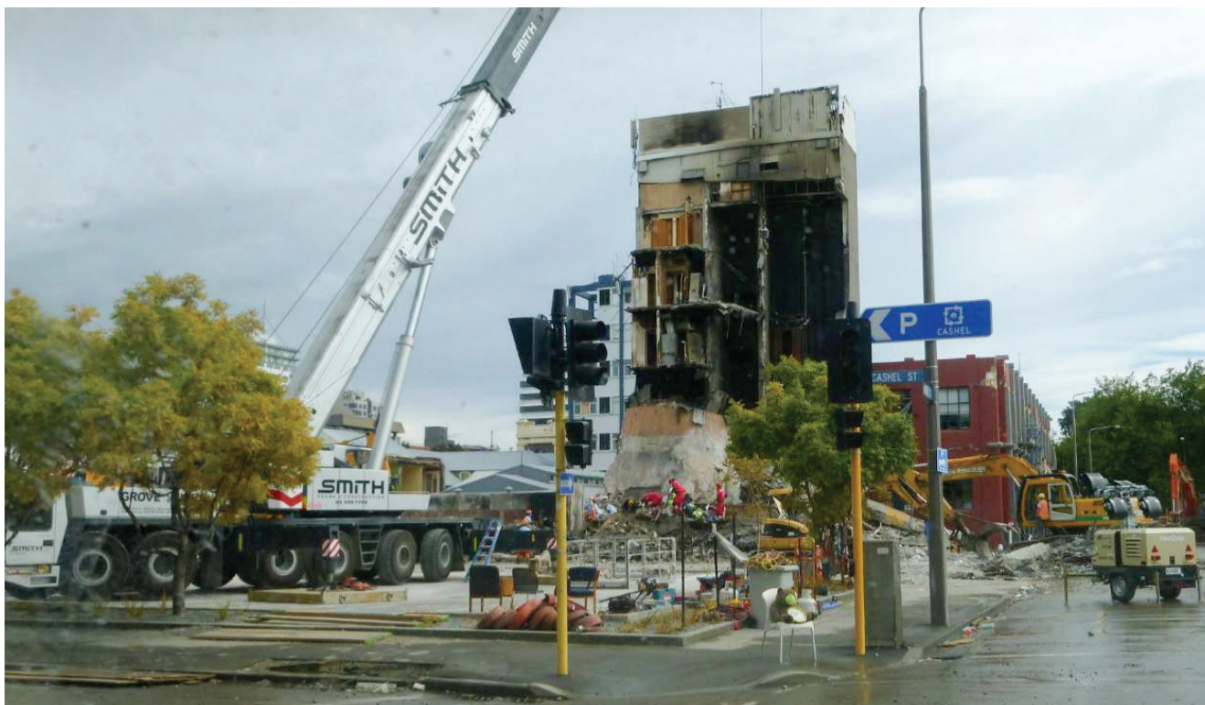
The collapse of the CTV building 10 years ago left a gaping hole in the Christchurch cityscape.
